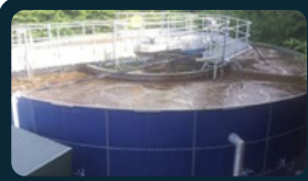
Activated Sludge Treatment
