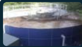
Activated Sludge Treatment
