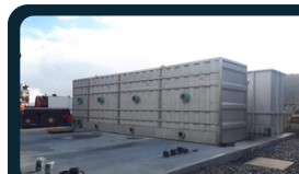
Rapid Gravity Filters
