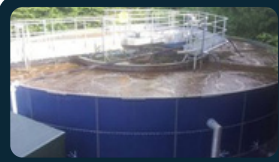
Activated Sludge Treatment
