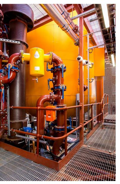
The units to connect the buildings were bespoke substations, designed and specified in conjunction with the designers, 3D models, built and delivered as pre-fabricated units and the Sondex PHE were also used elsewhere in the system as separation of circuits. The involvement in the project for Danfoss, was 4 years in total, from early design, through to contractor installation and commissioning. It is expected that the scheme will continue to phase 3, with further buildings connected.
